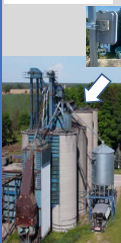
Installation of 60 GHz Network Installed In-Service Sept. 21, 2020
