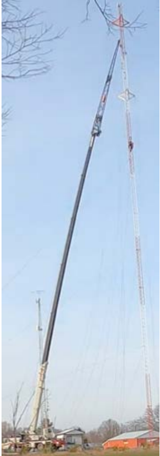
New 250' Tower Build - Completed Dec 2020
