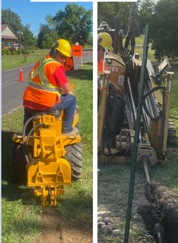
Installation of 4 km Optical Fibre Ring Completed Mid-January 2020 In-service End-November 2020
